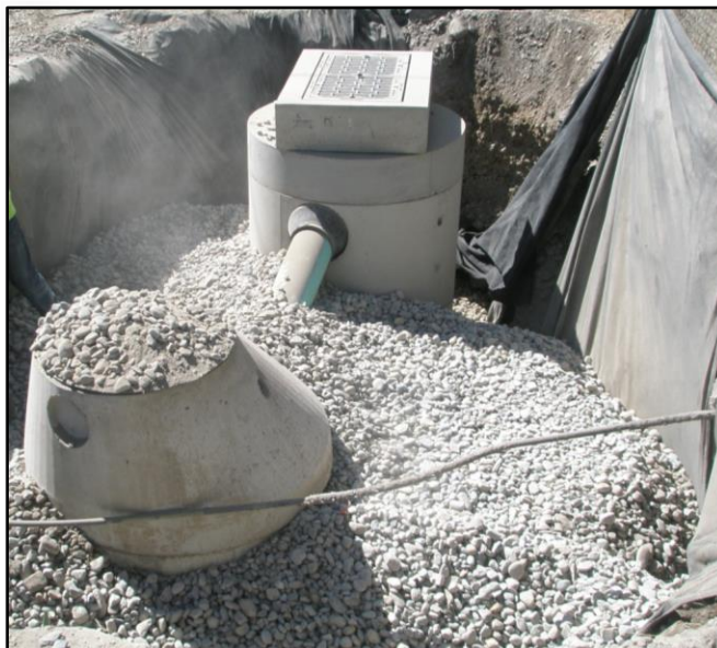
PICTURED: NEW DRYWELL AND TYPE II CATCH BASIN
