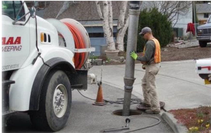
PICTURED: CONTRACTED STORM DRAIN CLEANING SERVICE OF A DRYWELL ON A RESIDENTIAL STREET
