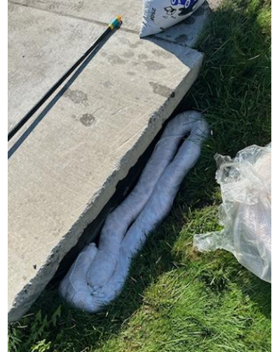
PICTURED: OIL BOOM PLACED TO PROTECT SWALE FROM OIL SPILL.
