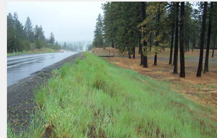
Dispersion BMPs allow runoff to infiltrate over a large area
