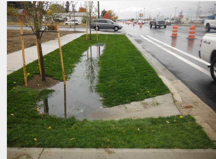
Bioinfiltration swale collecting stormwater road runoff
