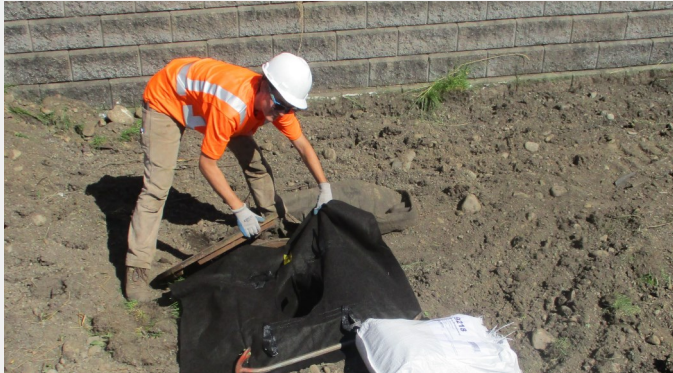
Catch basin insert installed during construction
