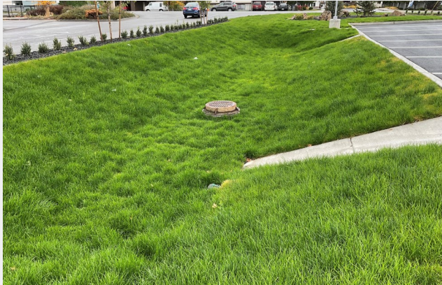
Bioinfiltration swale in Spokane Valley
